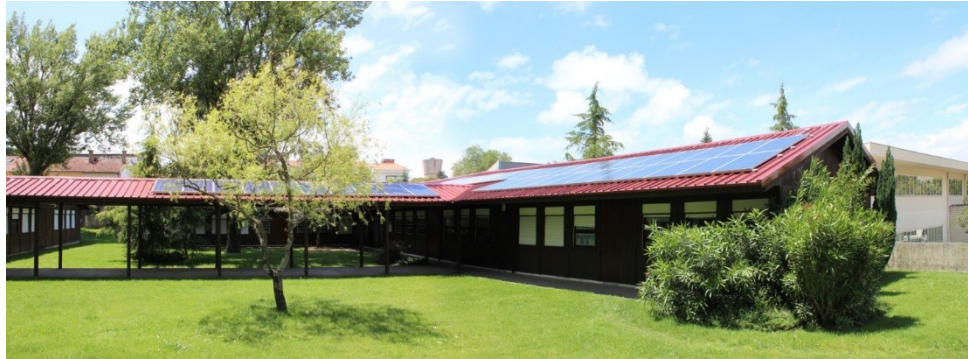
GECAD's Building N
